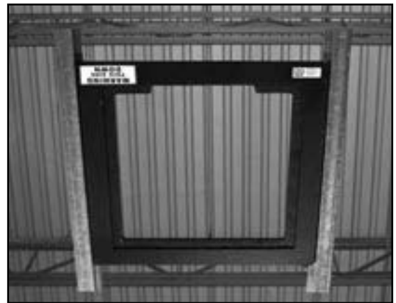
Figure 4: PIR installed on steel furring channel prior to drywall being placed.
